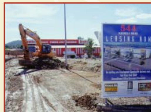
Macgregor Property, Building 1 construction and leasing campaign underway
