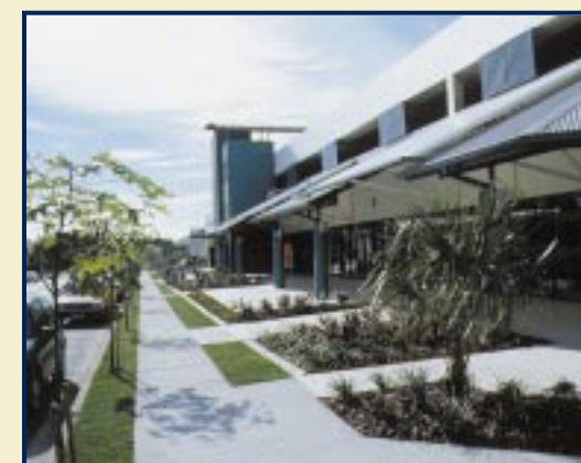
Harries Road aspect of the completed Coorparoo property
