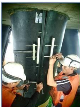
HDPE Jack Installation
