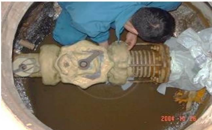
STACwrap UW - Underwater Petrolatum Tape using Non-woven, stitch-bonded, synthetic fabric carrier
