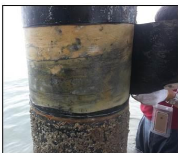
Installation of STACwrap on steel pile – 8 years ago (2007)
