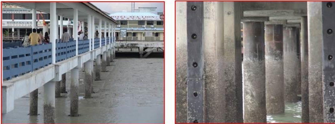
Piles After Installation of Corrosion Protection
