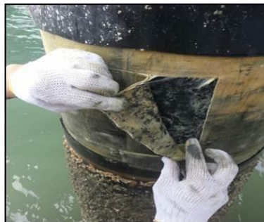
Cutoff Section of STACwrap – Inspection on March 2015
