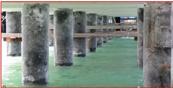
Coating of Steel Pile
