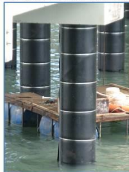
Jetty Steel Piles After Installation of Corrosion Protection
