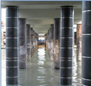
Jetty Steel Piles After Installation of Corrosion Protection
