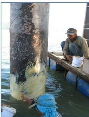
Jetty Steel Piles After Installation of Corrosion Protection
