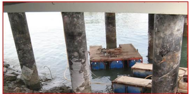
Installation of Jackets and Straps
