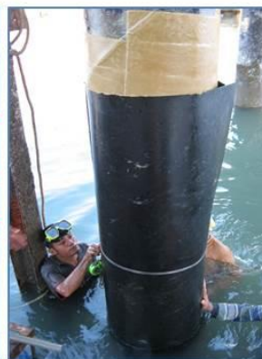
Installation of Jackets and Straps
