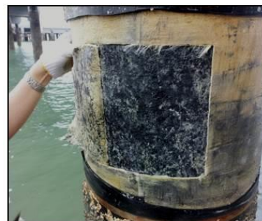
Steel Pile Surface is in good condition - (March 2015)
