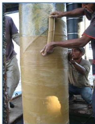
Jetty Steel Piles After Installation of Corrosion Protection
