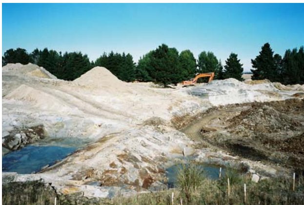
This photo relates the new trench excavation (to be under the perimeter of the TSF containment wall) to the location of the original impoundment wall (and the revealed overflow containment provision of 1899, at left).
