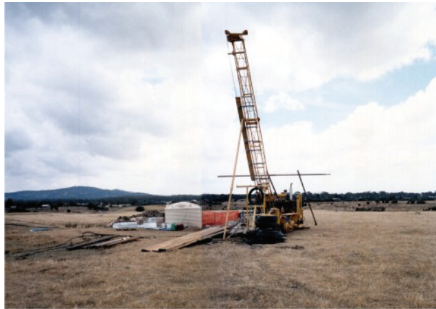
PHOTO 1 - View from east, rear (looking west)
